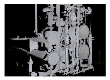
Two registered scans viewed together of a set of heat exchangers and associated piping within a refinery. Image courtesy Summit Engineering and Design.
